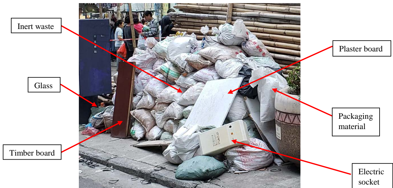
Figure 5.5 Site visit at Site E– Single Residential Building – Tak Shing Mansion
