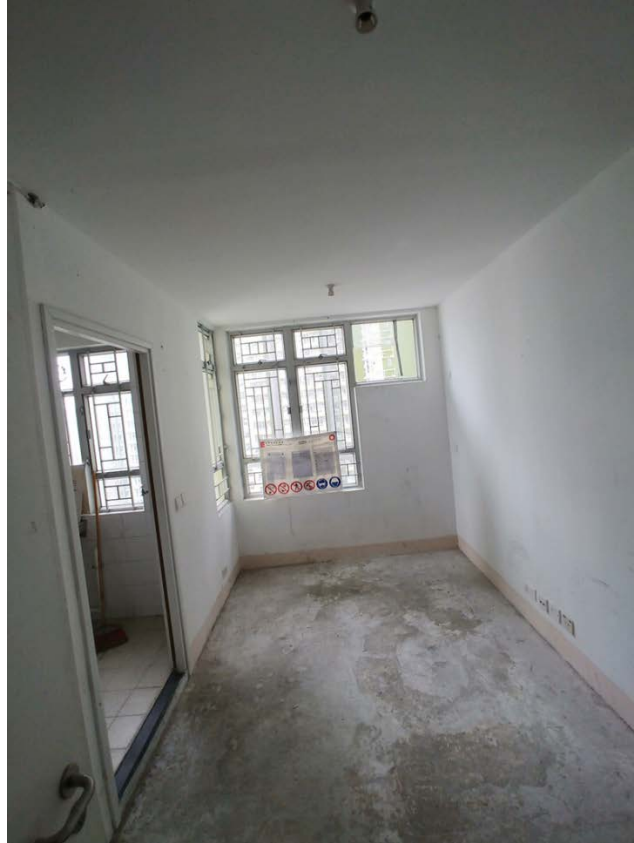
Figure 5.4 Site visit at Site D - Public Housing Estate 2 – On Tat Estate
