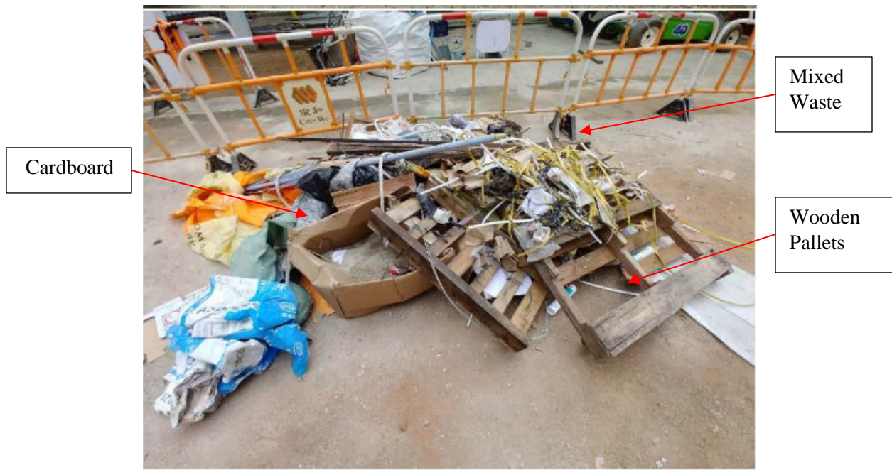
Figure 5.3 Site visit at Site C - Hospital – Hong Kong Buddhist Hospital
