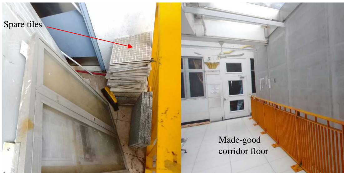
Figure 5.1 Site visit at Site A - Religious Buildings – Sikh Temple
